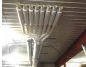
A turbine fan forces fresh air into a system of corrugated tubing encased inside a 20-ft. ventilation duct
