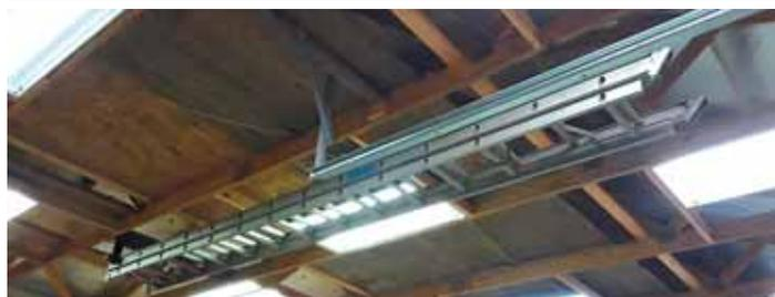
Extension ladder is suspended horizontally below shop loft when not in use, and is hinged at one end. It can be lowered to floor by releasing a rope tied to a boat cleat mounted on shop wall.
