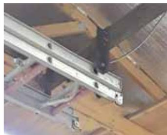
Upper end of ladder hinges on a pipe that runs through ladder’s top rung.
