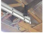
Upper end of ladder hinges on a pipe that runs through ladder's top rung.
