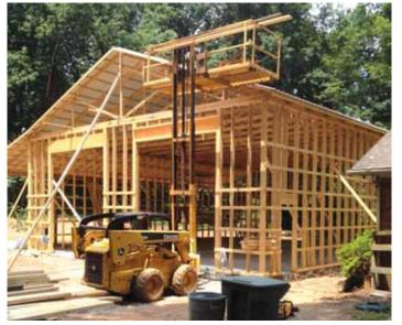
Industrial forklift mast attaches to skid loader arms and can be fitted with a 12-ft. long metal basket that slides onto the forks.
