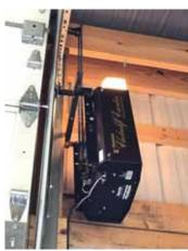
Larry Wood gained more overhead room in his shed by converting a standard overhead garage door opener to a side-
