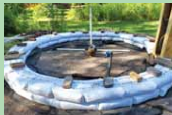
A raised tamped gravel pad was installed before walls were built (left). Cellar's roof plate is covered by a heavy rubber tarp to provide a watertight seal.
