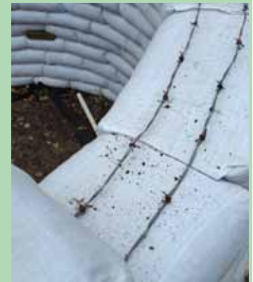
Rovig filled sandbags with dirt and then stacked them like bricks to form cellar's walls. Two rows of barbed wire between wall layers keep bags from slipping apart.
