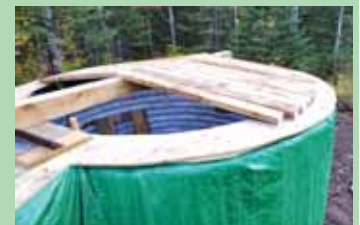
A raised tamped gravel pad was installed before walls were built (left). Cellar's roof plate is covered by a heavy rubber tarp to provide a watertight seal.
