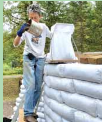
Rovig filled sandbags with dirt and then stacked them like bricks to form cellar's walls. Two rows of barbed wire between wall layers keep bags from slipping apart.
