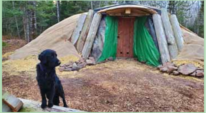
Sherry Rovig used earthbag construction to build this root cellar. The 10-ft. dia. room with 6-ft. walls is topped by a wooden roof insulated with dirt.
