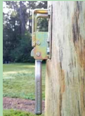
“Drop” gate latch consists of an upper catch latch and a hinged, 2-pronged fork. Pulling the catch latch up drops the fork, allowing gate to swing in either direction.
