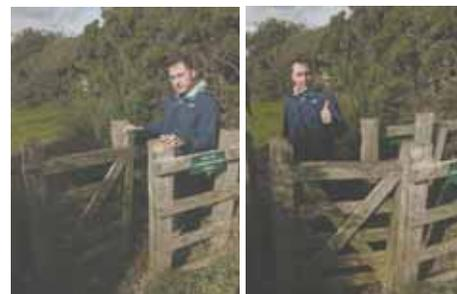
Pass-through gate swings back and forth inside a U-shaped set of fence panels, leaving just enough room to pass.
