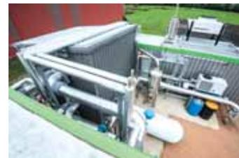
Photo above shows exterior view of a smaller modular manure digester set up by Brian Langolf. System produces biogas that fuels a 64 kW CHP generator.
