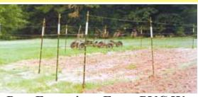
Beggs used short lengths of pvc pipe and post to make his 6-ft, high electric fence even higher.
