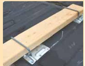
Boards slide into rectangular metal brackets.
