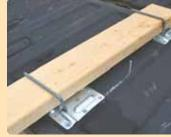
Boards slide into rectangular metal brackets.
