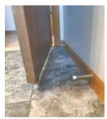
Small magnets mounted on door and doorstop keep bathroom door open.
