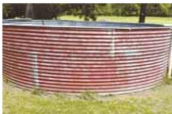
Margaret Adams bolted steel grain bin panels together to make this 24-ft. dia. swimming pool.
