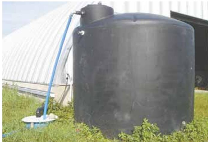
Rain water from Quonset building is collected by an 80-ft. eavestrough that feeds into a sump at end of building. From there it's pumped to a 3,000-gal. holding tank.
