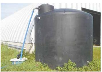
Rain water from Quonset building is collected by an 80-ft. eavestrough that feeds into a sump at end of building. From there it's pumped to a 3,000-gal. holding tank.
