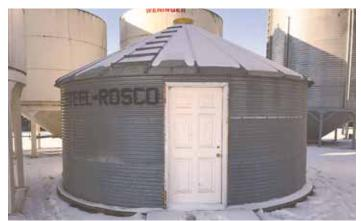
Leland Heuchert made this storage shed mostly from used bin parts. He assembled 3 rings and a roof from a 19-ft. bin, then installed a used door purchased online.
