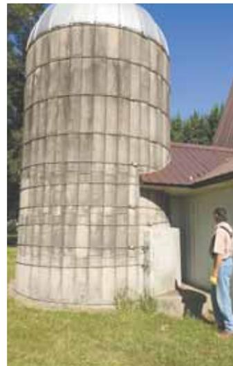
**To rebuild his silo for farm storage, Rinke cut a new walk-in door into the staves, then poured 3-ft. high by 8-in. thick concrete "wings" on both sides of it. Silo's lower 2 band rings are embedded in the concrete.**
