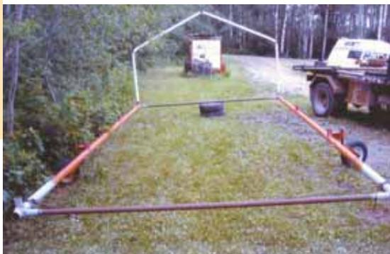
Arnold Bergesen used 3-in. dia. pipe and caster wheels to build a frame for his 10 by 20-ft. plastic storage shelter. Frame has pockets on the sides and corners that the shelter's hoops pin onto.
