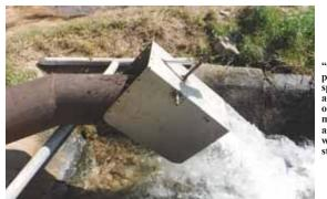
"Coon preventer" spout automatically opens with moving water and closes when water stops flowing.
