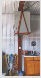
Marvin Boehm, Sherwood, Ohio: "I have a small farm shop where I keep my restored tractors and other farm stuff. I like some heat in winter but only on an intermittent basis. I bought a used 'downflow' gas furnace from a contractor who was replacing all the units in an apartment house. It mounts in an angle iron frame that I welded together and then suspended from a steel beam across the top of the shop.
