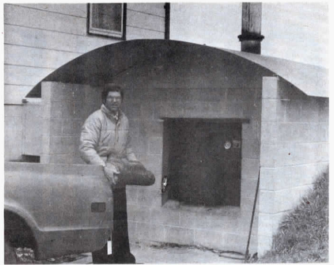
Ross Olson's home-built outdoor furnace stores enough heat to last 2 days in his 2,800 sq. ft. house.
