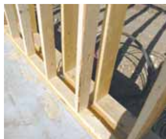
Double stud walls have a 3-in. space between them for a total rating of R-43. Photo at right shows plumbing for in-floor heat.
