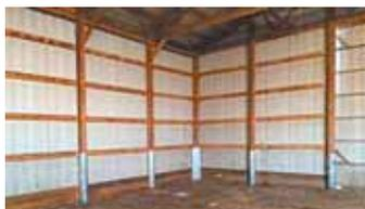
**Made of galvanized steel, the 6-ft. long, 3-sided Strong Way Sleeve is designed to reinforce existing wood posts that have decayed at ground level and below.**
