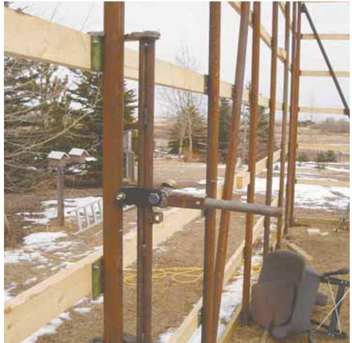
"Tensioner tool" works like a cam to slightly pre-bend pipe before McNaughton welded on it. It consists of a 3-ft. length of welded-together double pipes with steel hooks welded on top and bottom, and a pipe handle with a steel yoke at the end. (Photo illustrates use on pipe that has already been welded.)
