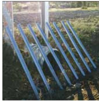
"It keeps trash from catching on wire fencing and culverts," says Joe Pacheco about his "pipe fence" kit. It consists of a reusable metal template that helps drive pipes that work with the flow of water.
