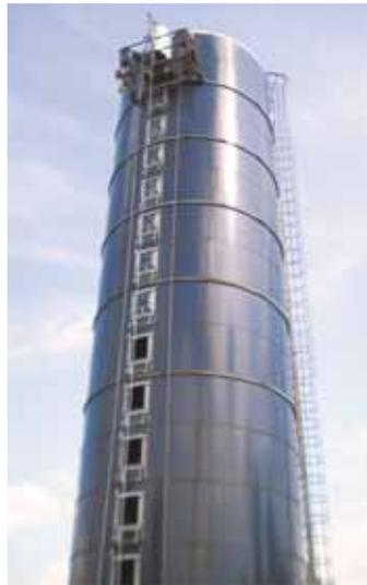
Doors and a chute are added to outside of Harvestore and a top silo unloader installed.
