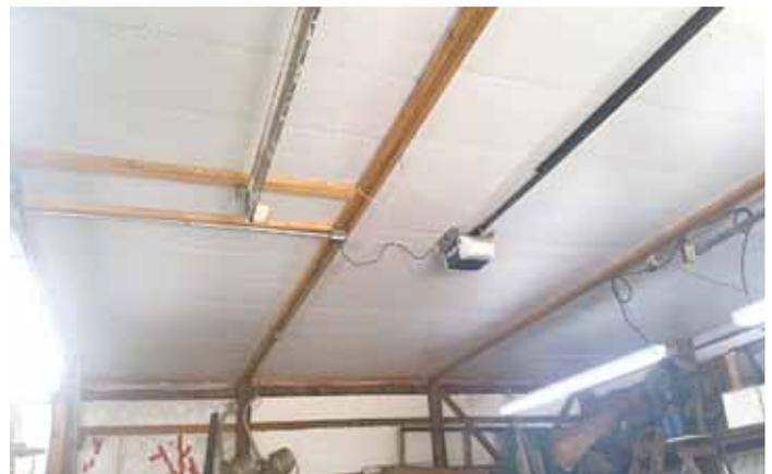
Brauer installed 2 by 2's at the bottom of the trusses in his shop and laid in garage door panels, then added 3 1/2 in. of insulation on top that's covered with Tyvek.
