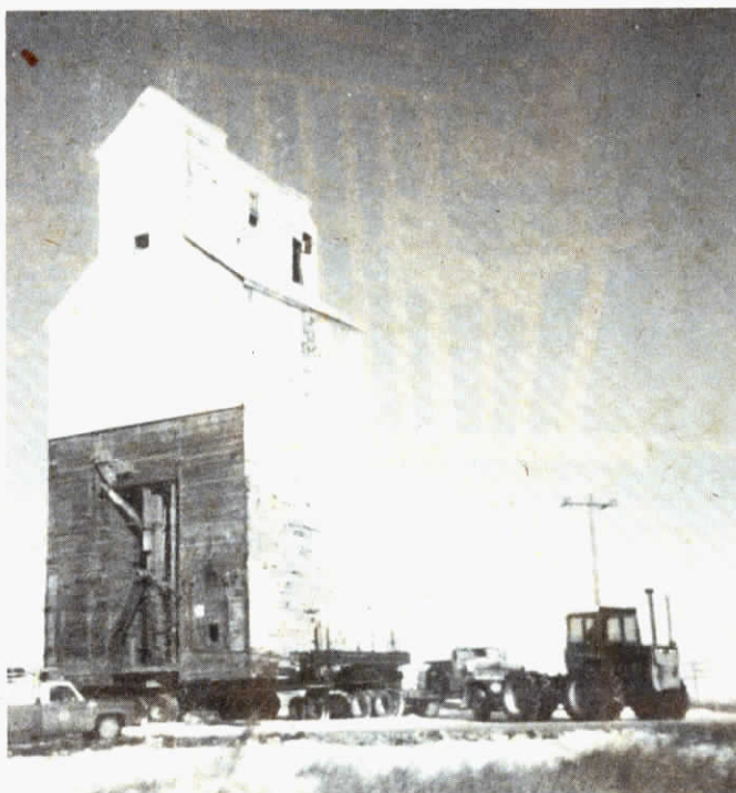
During elevator moves, Digney always has at least one Caterpillar and a couple big tractors standing by to help skid dollies around corners.
