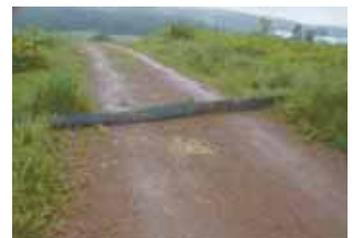
A length of rubber conveyor belt is bolted to 2 by 6-in. treated boards, that are then buried in the ground. The belting diverts water from road surface.
