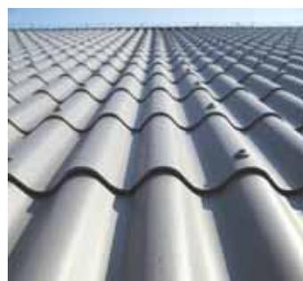
High density fiber cement corrugated roofing sheets wick moisture from inside buildings to the outside.
