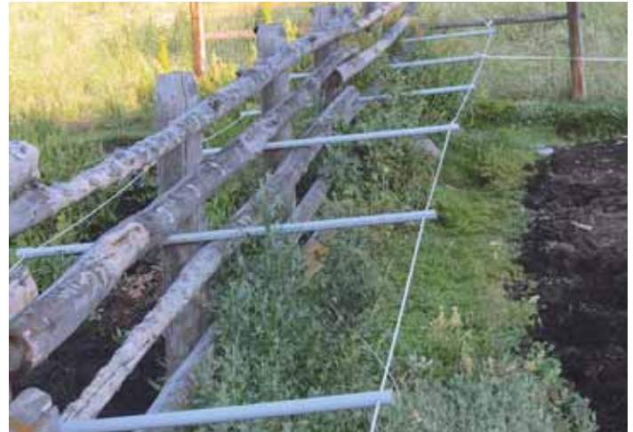
Pvc conduit "insulator arms" hold a single strand of electric fence wire to keep horses from getting close enough to chew or rub on wooden fence rails.
