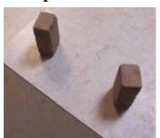
When Meihak tiled his shop floor, he used only a small amount of adhesive under each tile so he can easily replace any that become damaged.
