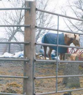
Horse-high fence is constructed with 16-ft. sections of pipe. Pipe panels attach with U-shaped brackets to wooden fence posts.
