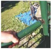
Latch end of gate is fitted with a retractable bolt contained in a round tube.
