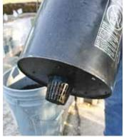
Plastic net filter cup is inserted into hole cut into bottom of each bucket, to draw water out of rain gutters
