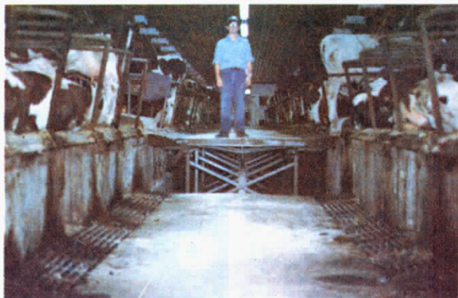
But, at milking time, the entire 240 ft. center aisle drops 28 in., and restraining bars drop behind cows.
