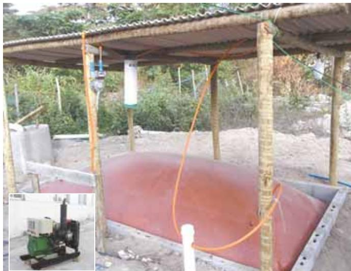
A Swiss company works with individuals who want to build biogesters on their property. Methane expands the top of flexible rubber bladder and is released through a flexible line. Biogesters can be used to operate engine-powered generators.
