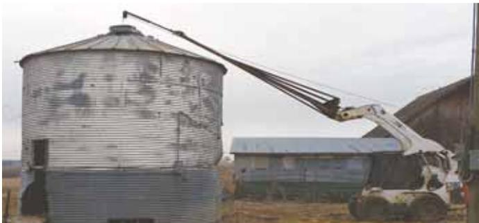
He made a 16-ft. long boom for his skid loader and used it to lift bin’s roof and top ring of panels.
