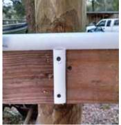
Pvc "butt joint protector" locks fence boards together at the joint to keep horses from pulling them off.
