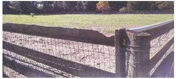
Pvc cap (at right) slips on over worn fence board and attaches with countersunk screws spaced 16 in. apart.
