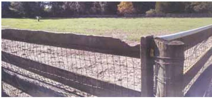
Pvc cap (at right) slips on over worn fence board and attaches with countersunk screws spaced 16 in. apart.
