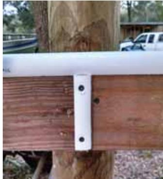
Pvc "butt joint protector" locks fence boards together at the joint to keep horses from pulling them off.
