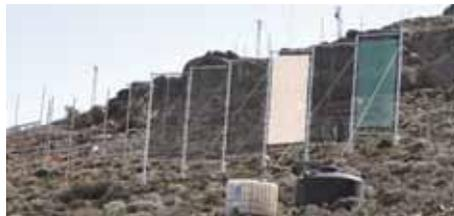
Fog that condenses onto mesh nets set up on hillsides is piped up to 5 miles away for use by local villagers.
