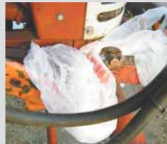
**Gary Swensen, Yankton, S. Dak.:** "Whenever I have to do spot painting on equipment, instead of using masking tape I just use old plastic grocery bags. It's easy to tuck the bags into tight places, and they can be left on indefinitely without leaving any sticky residue like with tape. And after the bags dry out they can be reused. The photo shows how we recently used plastic bags while painting the mounting brackets on our front-end loader."
