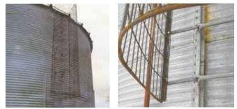
Lester Adelman used a round corn crib panel to make this safety cage that surrounds the ladder on his grain bin. Brackets run from ladder to angle iron attached to cage.
