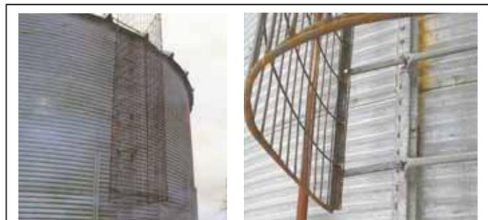
Lester Adelman used a round corn crib panel to make this safety cage that surrounds the ladder on his grain bin. Brackets run from ladder to angle iron attached to cage.
