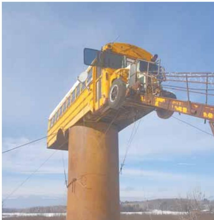
**Jesse Kauffman's one-of-a-kind deer stand is a roomy 72-passenger bus welded on top of a 28-ft. gas tank standing on end, anchored 10 ft. deep into the ground.**
