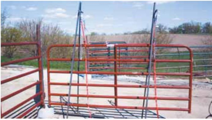
Two tall A-frame hangers, fitted with a chain and ratchet strap, are used to make sure hanging gate stays level as it's being welded to sleeve on post.
