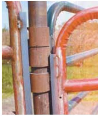
Round metal sleeves on heavy metal post serve as hinges that allow gate to be rotated 360 degrees. Foster attaches a 2-in. channel iron to gate and then welds it to sleeves. Up to 3 gates can be attached to the same post for making pen dividers.
