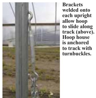
Brackets welded onto each upright allow hoop to slide along track (above). Hoop house is anchored to track with turnbuckles.
