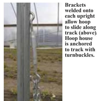
**Brackets welded onto each upright allow hoop to slide along track (above). Hoop house is anchored to track with turnbuckles.**
