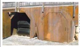
Gary Witter and his brother Danny turn old fuel tanks into various storage units. Tank can be left above ground or buried.
