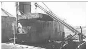
Farm Fans dryers are the simplest, most effective dryers ever built. The only moving part is a pto-driven fan.
