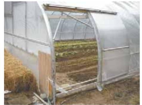
**Norris needed cross framing on ends of tunnel for structural integrity when moving the building, so he moved the entry door to the side.**
